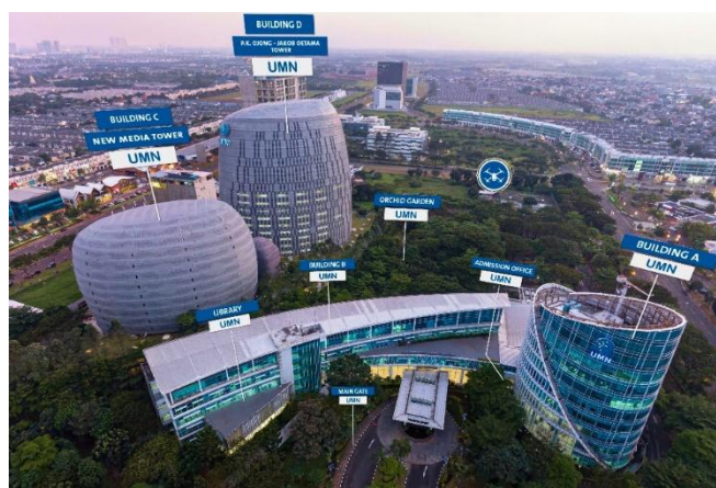
Figure 1. Four buildings in UMN [15]
